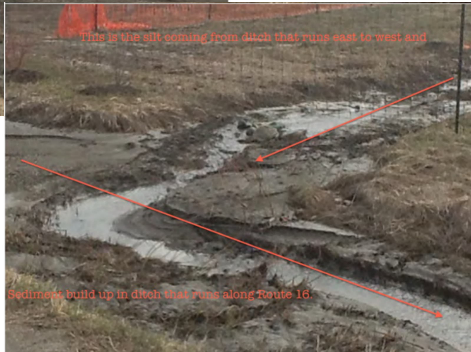
Silt along route 16. Note culvert located on Northern property drive.
